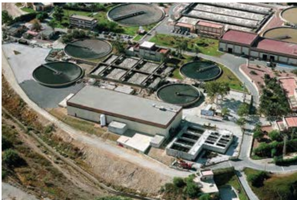
A bird's eye view of the Alicante tertiary treatment facility in Spain. The reverse osmosis membranes were selected as they would better handle the solids passing through the ultrafiltration membranes.
