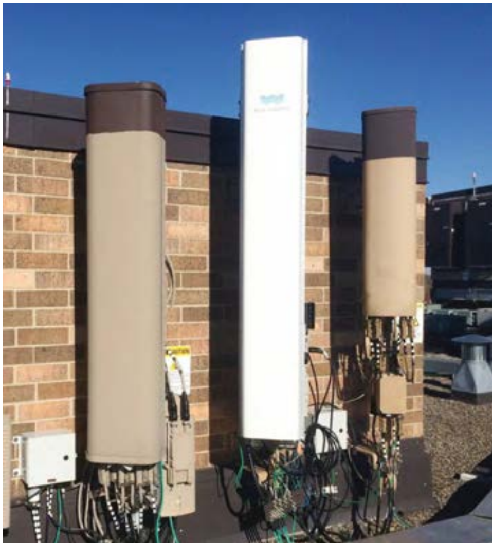
Massive Multiple input multiple output (MIMO) systems multiply radio link capacity using multiple transmission and receiver antennas via multipath propagation.
